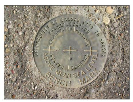
**Benchmark:** A benchmark is a permanent marker (usually a bronze disk) at a determined point that identifies a fixed location (elevation and horizontal coordinates) and is used as a reference point for surveys in its locality.
